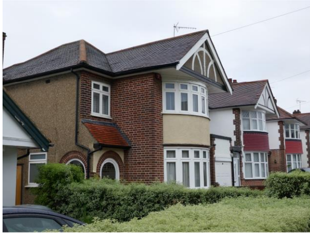
Appendix 4-B - photos of Suffolk Road
